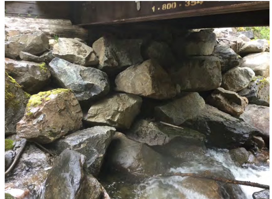
Left Bank Abutment when facing downstream
