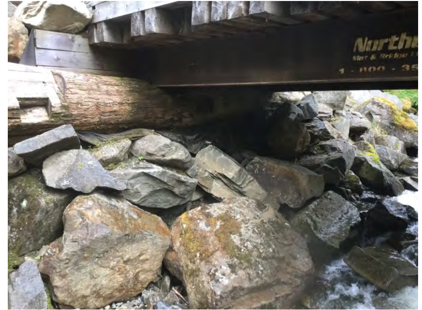
Right Bank Abutment when facing downstream
